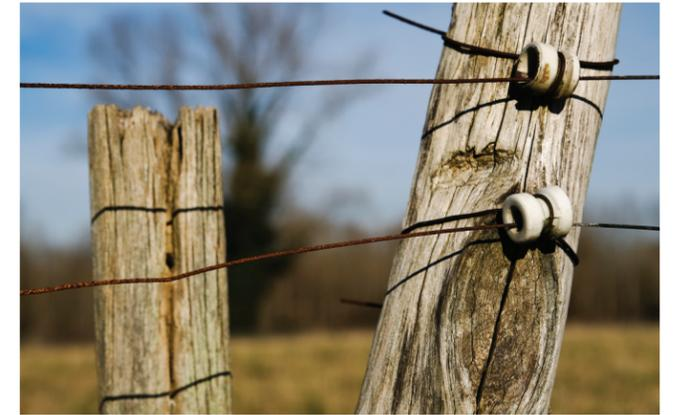
**Electric fences are specially insulated from the ground and can pick up an induced charge from transmission lines.**
