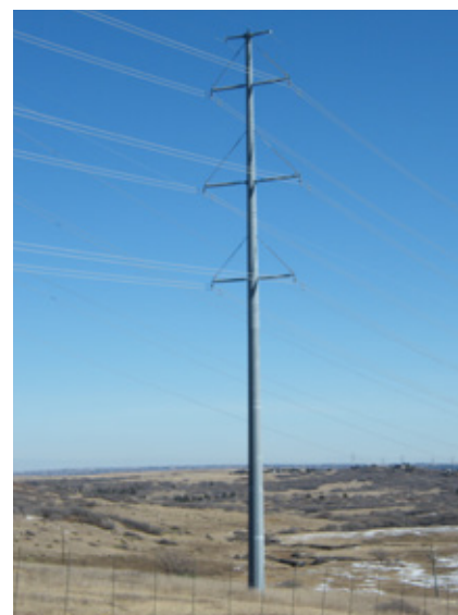
Single pole structures will be mostly used except for corner structures where multiple poles will be used.
