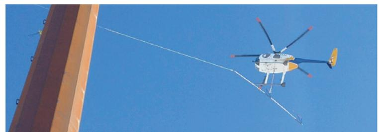
We will use a helicopter to assist in the stringing of conductor, which enables installation in difficult-to-access areas and helps protect sensitive environmental areas.
