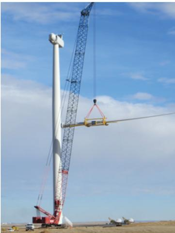
The first of three blades is lifted for attachment to the hub. Each blade is approximately 180 feet. They are being fabricated in Brighton and Windsor by Vestas.
