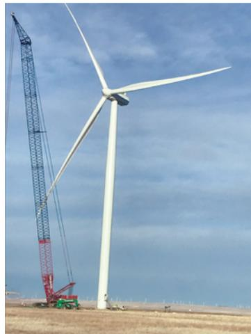
We erect the wind turbines using a 310-foot crane with a lifting capacity of 880,000 pounds. It requires up to 27 trucks to deliver all of the crane pieces to the job site.
