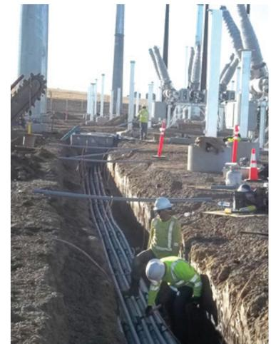
Crews install duct bank at the new Pronghorn Substation.
