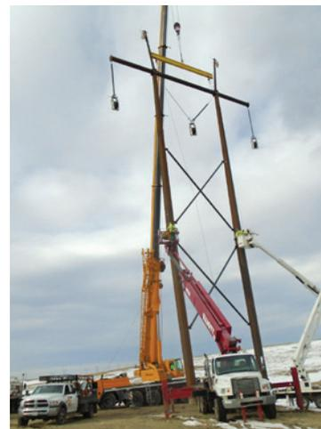
Transmission structures are 100 to 130 feet tall with a 150 foot right-of-way.
