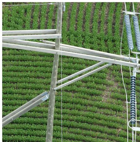
Data from a UAS mission in Minnesota shows a broken cross-arm on a transmission structure.
