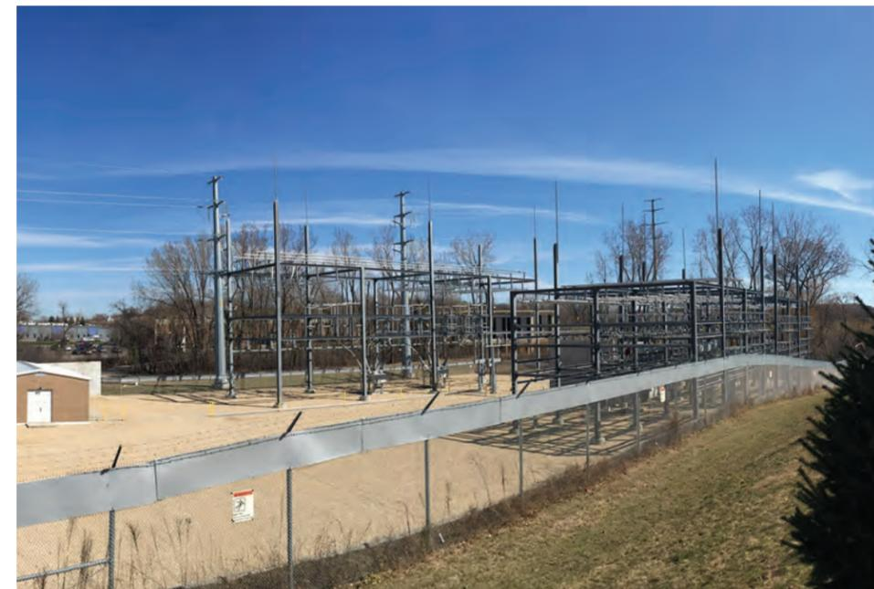
**Alternative C requires a new Pomerleau Lake Substation. A similar substation is pictured on the left. Substations change voltage and are interconnection points allowing energy to travel to your homes and businesses.**
