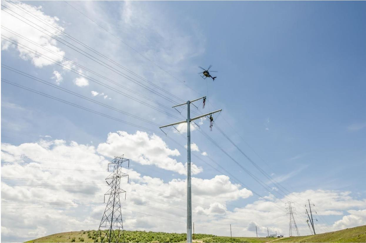
Xcel Energy used a helicopter to help crews in stringing conductor lines on the Pawnee-Daniels Park 345 kV transmission line project in Aurora and Parker.
