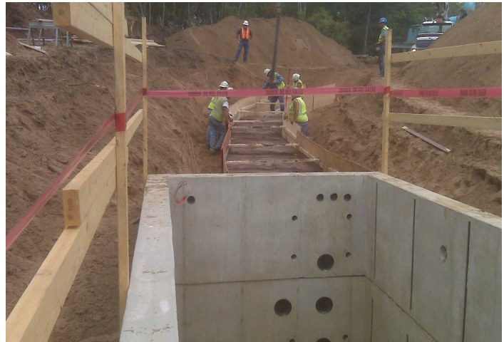
Crews work on an underground duct bank extending from a typical 8'x8'x24' vault
