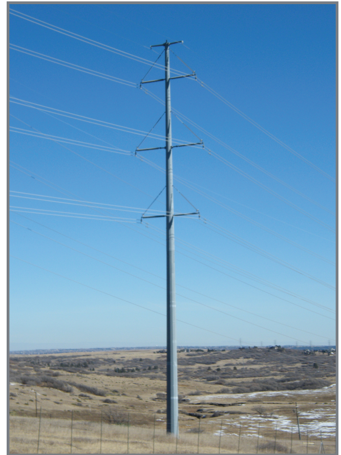
Construction on the Northern Colorado Area Plan includes single-pole steel structures ranging between 80 and 130 feet in height.
