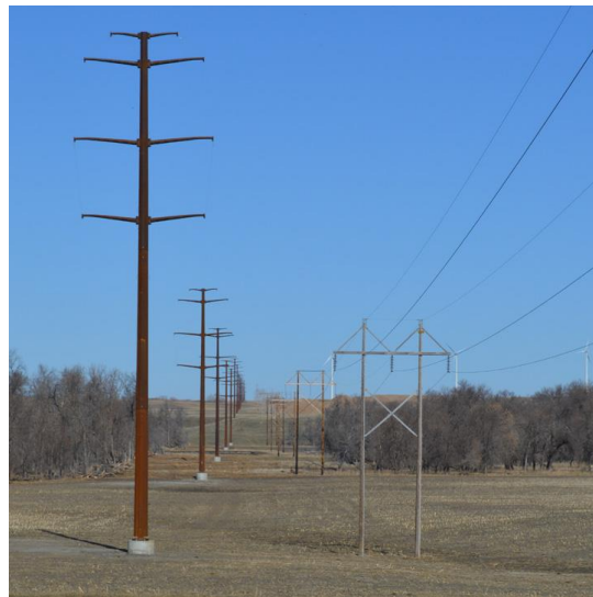
Single pole steel structures (left) were used on the new transmission line. The H-frame structures (right) will be removed later this year.
