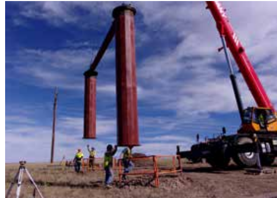
Structure setting is underway on portions of the project.
